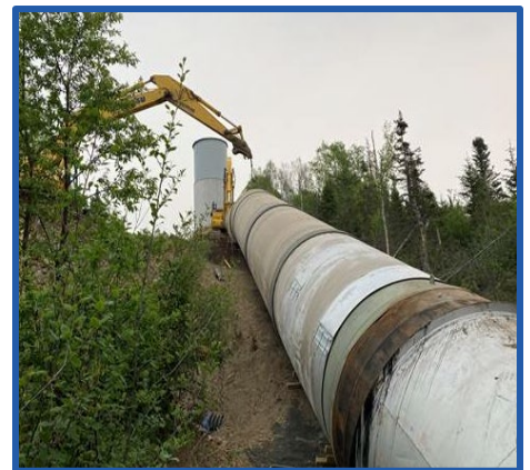
Newly constructed section of penstock at Sandy Brook hydro plant.
