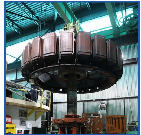
Rotor at Sandy Brook hydro plant being removed.
