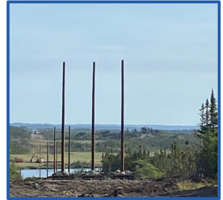
Poles installed on the second section of transmission line 94L.
