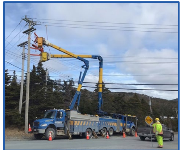
Traffic control set up for line operations work.
