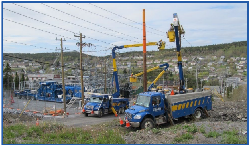
Work beginning at the Walbournes Substation in Corner Brook.
