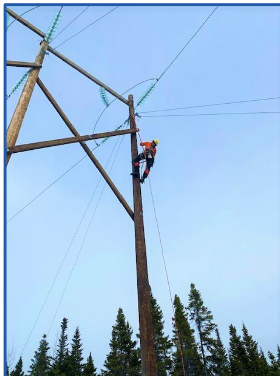
Crews completing maintenance on transmission line 363L in Western region.
